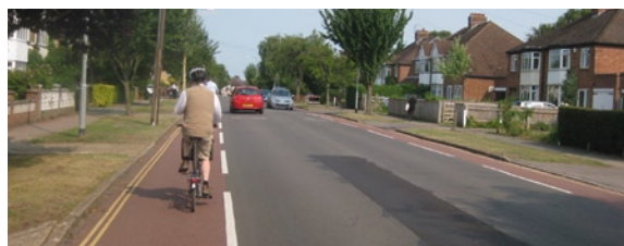
Centre line removal, Cambridge
