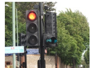
Green cycle pre-signal gives 5 seconds head start for cyclists, Examples in Brighton, York and Cambridge (requires authorisation)
