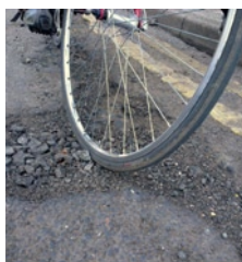
Repair damaged surface
