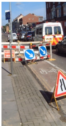
Provide for cyclists at roadworks
