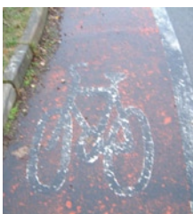
Facility ineffective due to poor maintenance
